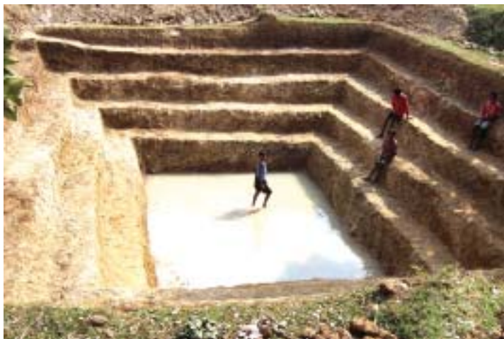
Excavation of tanks with 1:1 slope.
