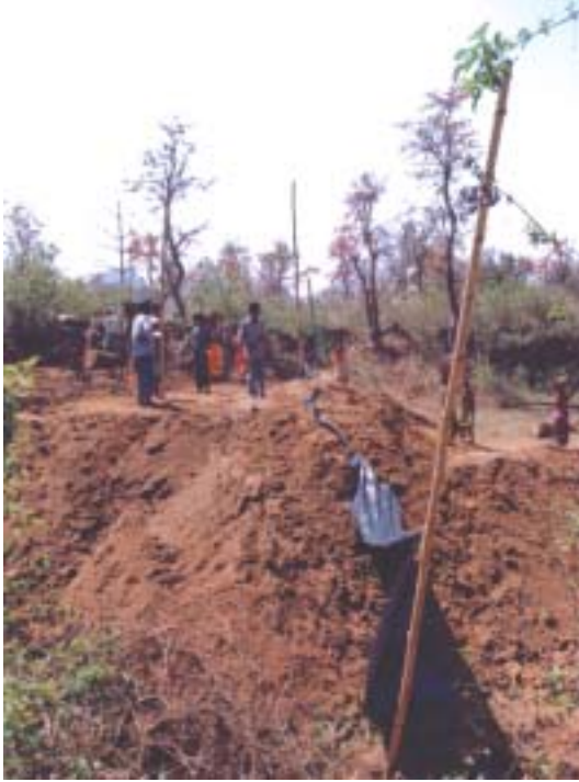
Providing water line for agriculture land.
